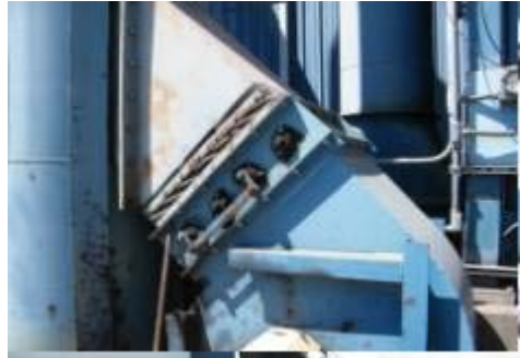
above pic shows motorized louvered assembly on dust collector fan.
